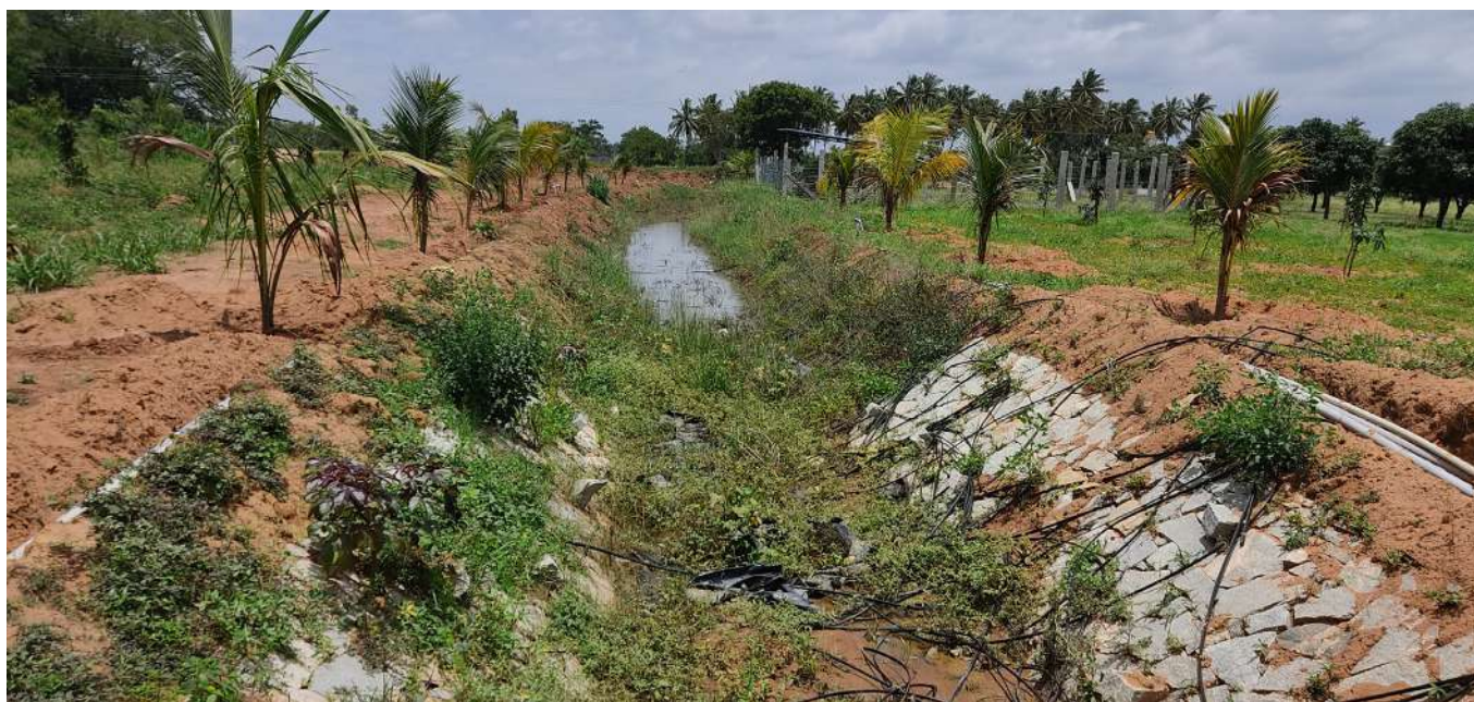
Channel development in Muduvadi GP
