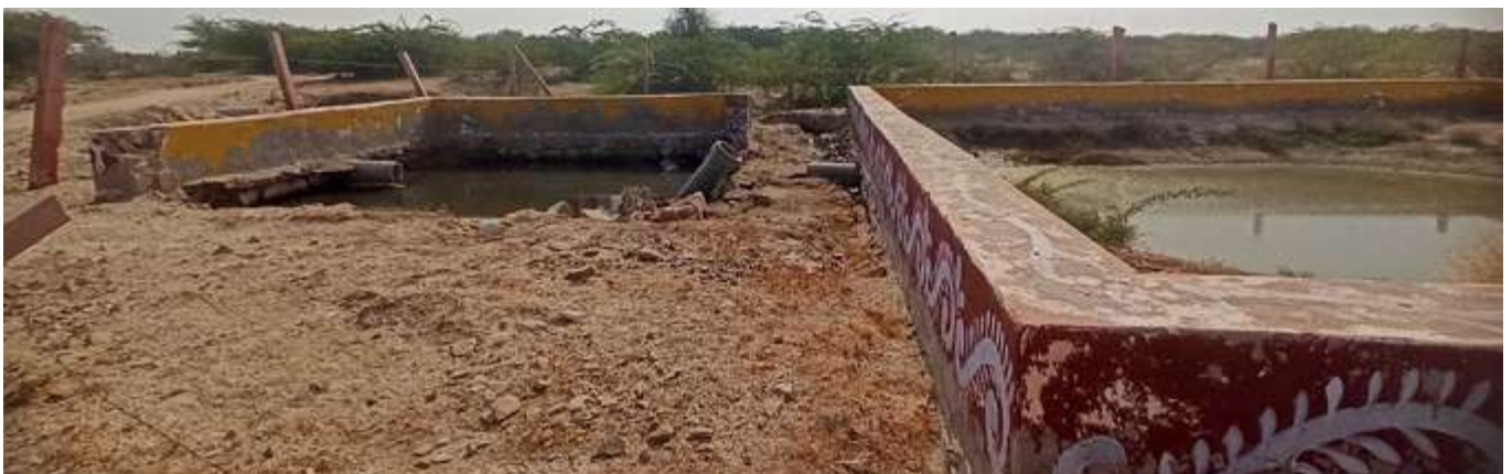
A portion of treatment system damaged due to heavy rains in Bhatinda Village, Luni Block, Jodhpur District,
