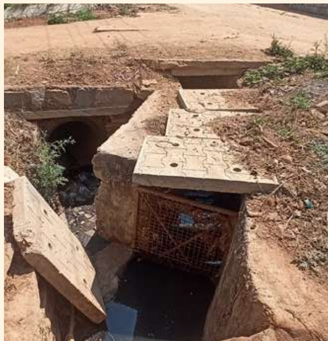
Separate diversion channels of stormwater and greywater in Muthur Village, Sidlaghatta Taluk, Chikkaballapur District, Karnataka.
