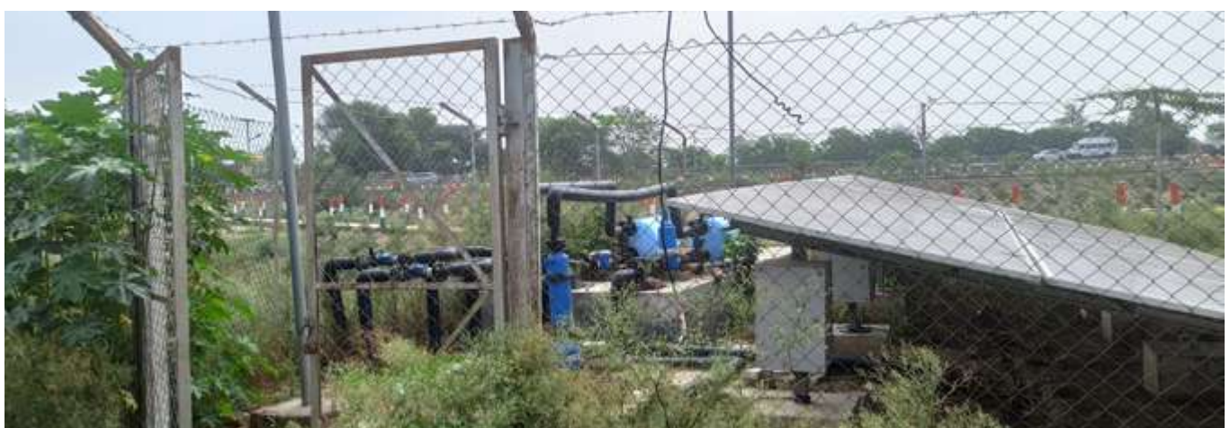
Solar powered pumping of treated greywater in Samana Bahu Village, Nilokheri Block, Karnal District, Haryana.
