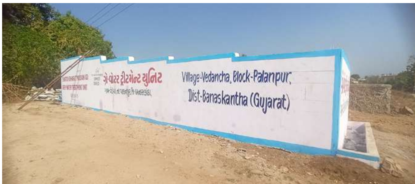
DEWATS system in Vedancha Village, Palanpur Block, Banaskantha District, Gujarat.
