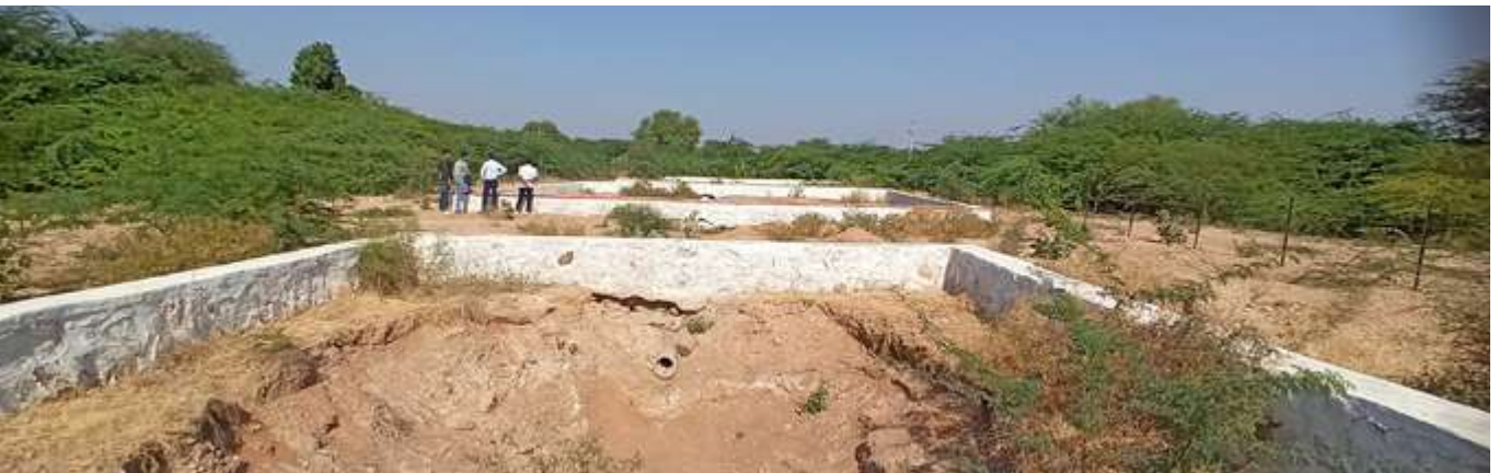
Treated greywater doesn't reach the Maturation Pond due to high evaporation rates in Sevaki Khurd village, Baori Block, Jodhpur District, Rajasthan.
