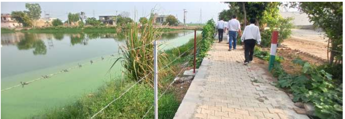
Community walking path along side of the constructed wetland in Barani Khalsa Village, Nilokheri Block, Karnal District, Haryana.
