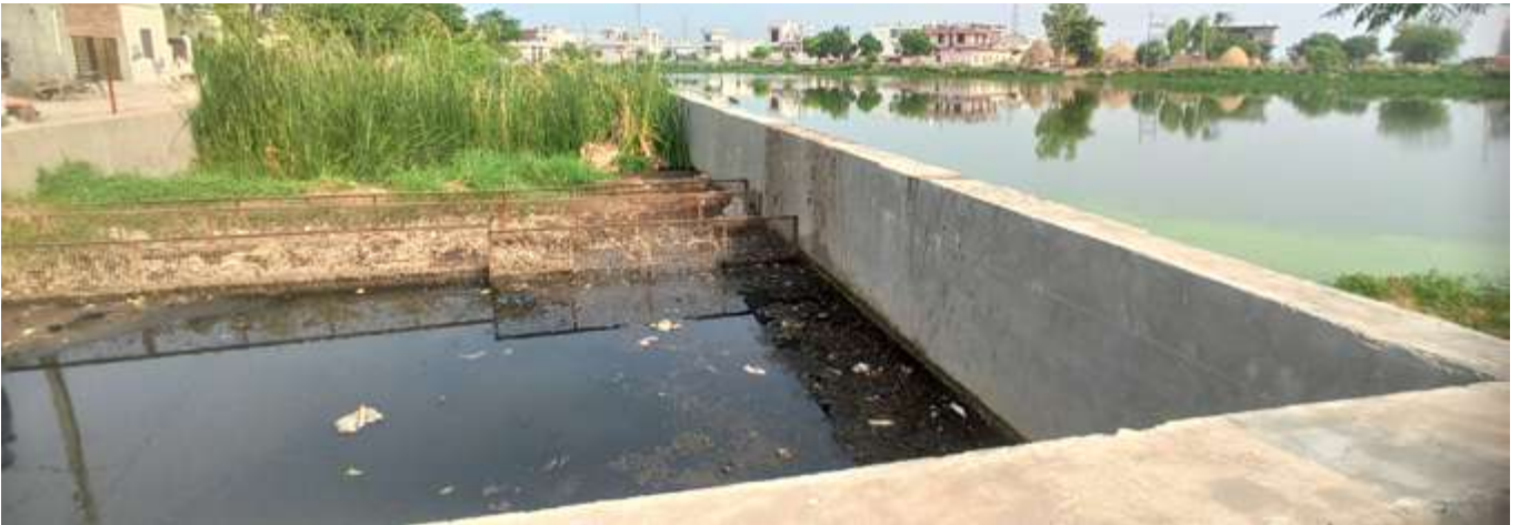
Stabilization Pond along with Vetiveria Zizanoides plantation as part of a treatment in a constructed wetland in Barani Khalsa Village, Nilokheri Block, Karnal District, Haryana.
