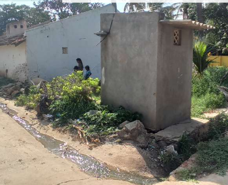
Greywater treatment system in Muthur Village, Sidlaghatta Taluk, Chikkaballapur District, Karnataka.
