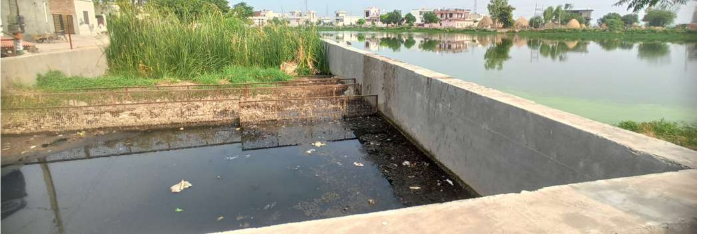
Stabilization Pond along with Vetiveria Zizanoides plantation as part of a treatment in a constructed wetland in Barani Khalsa Village, Nilokheri Block, Karnal District, Haryana.
