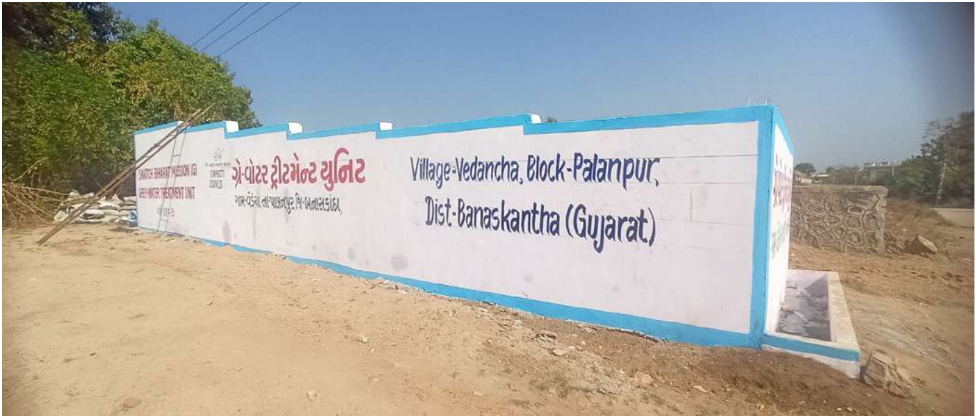
DEWATS system in Vedanacha Village, Palanpur Block, Banaskantha District, Gujarat.
