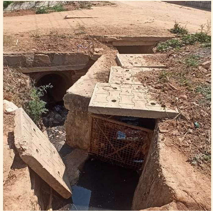
Separate diversion channels of stormwater and greywater in Muthur Village, Sidlaghatta Taluk, Chikkaballapur District, Karnataka.
