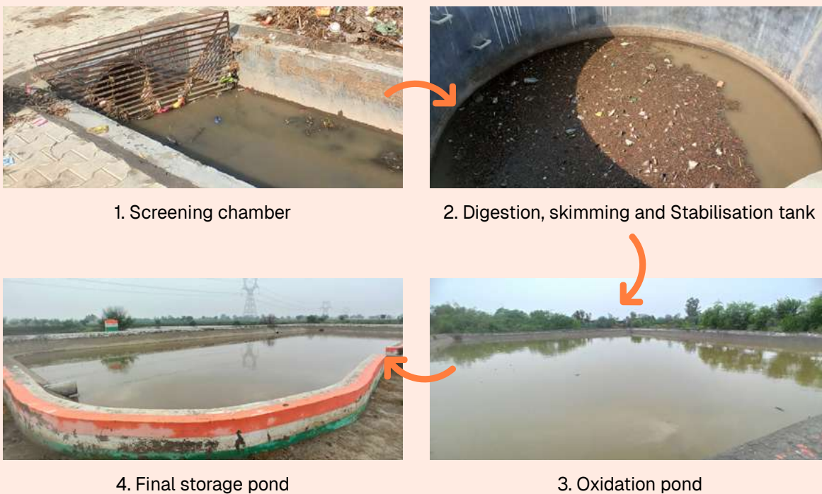
Figure 9: Schematic flow of steps involved in Waste Stabilization Pond (Thapar Model) treatment system.
