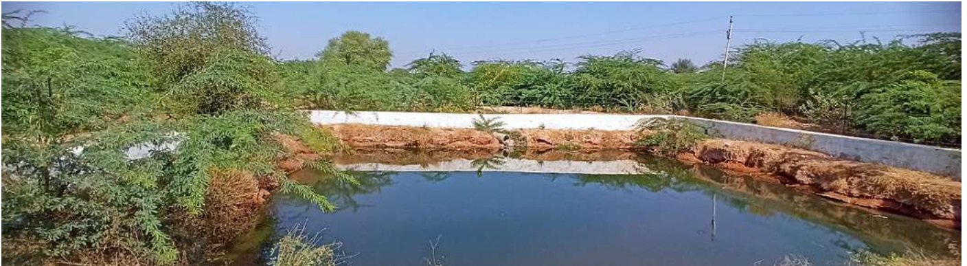
Waste Stabilization Pond in Sevaki Khurd Village, Baori Block, Jodhpur District, Rajasthan.
